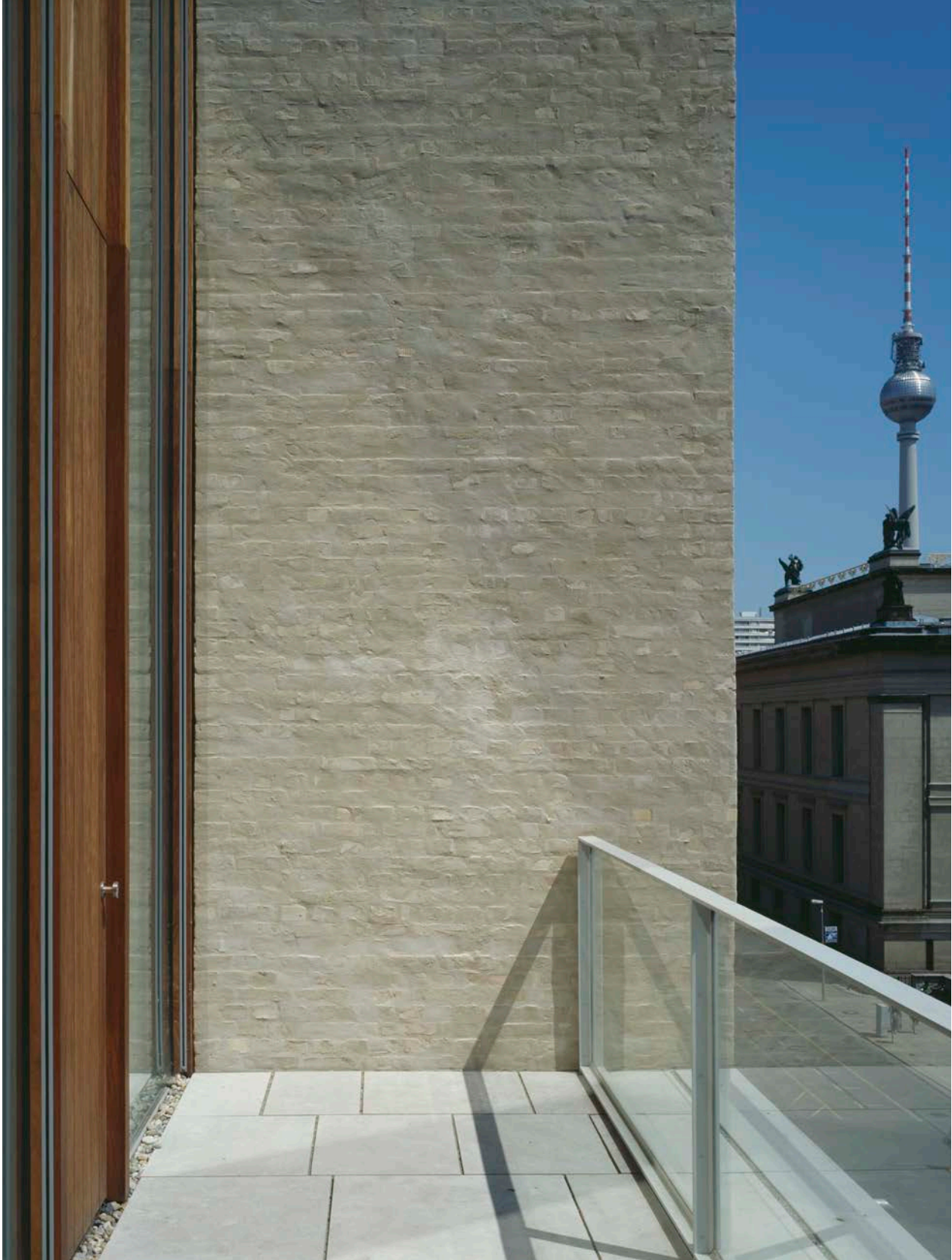
Gallery building Am Kupfergraben
